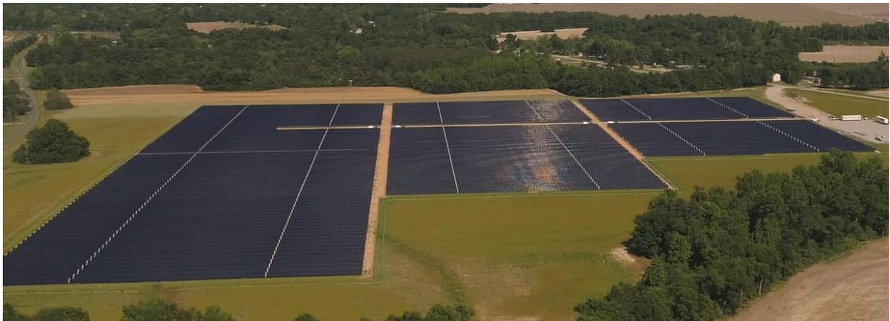
Nimitz Solar Farm, located in Jasper County, consists of more than 89,000 panels, each providing up to 120 watts of DC power for SCE&G's community solar program.
