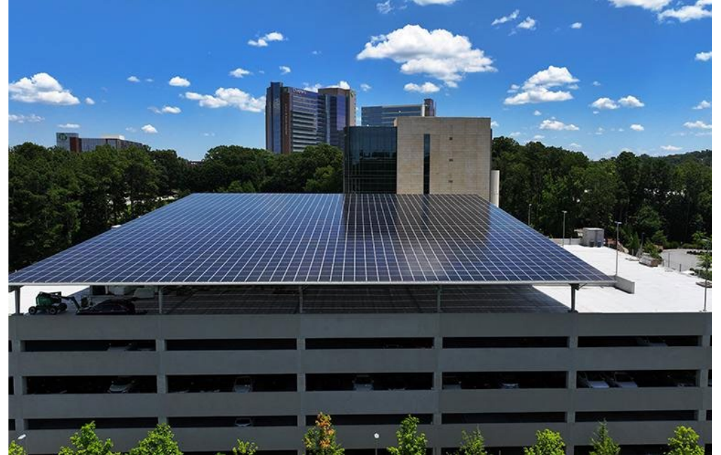
* Emory University Parking Garage Solar Canopy
