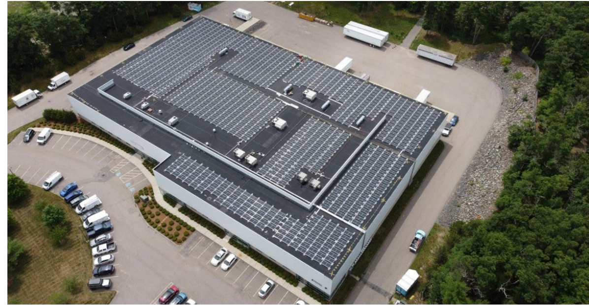
523kw System in Foxborough, MA GTR Engineering, Financing and Supplied
