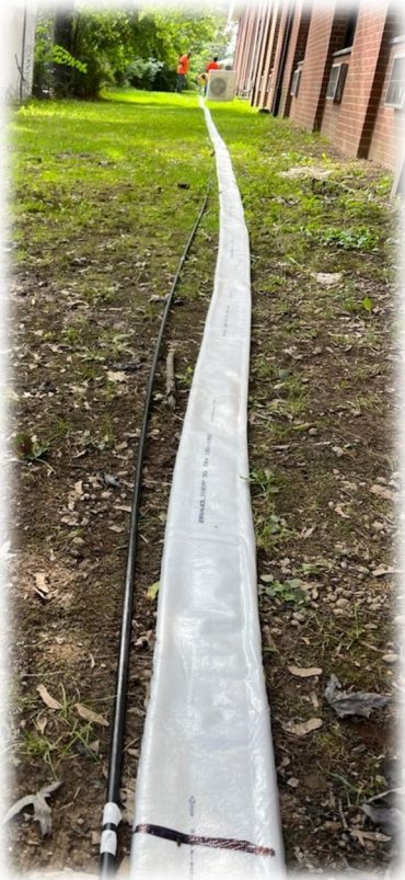
Liner Measured & Cut
